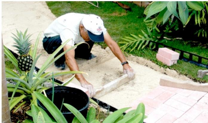
Kalihi's Dan Nakamatsu carefully levels sand before laying bricks in a service project to build a walkway at Phil Chun's house.
